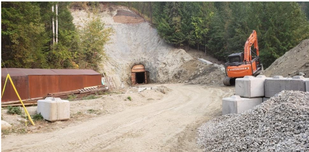
Photo of Kenville 257 Mine Level Portal and stockpile of crushed gravel for bedding (right).
