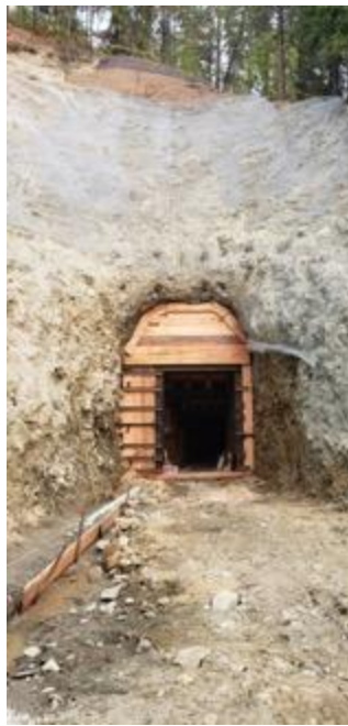
Photo of new entrance installed in Kenville 257 Portal.
