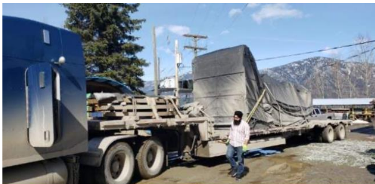
Long anticipated delivery of the Steel Sets for the New Portal Construction
